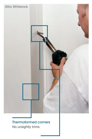
Heat welded joints
