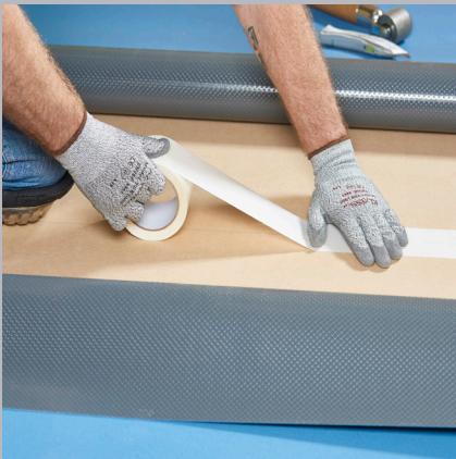
Tape perimeter and seams
