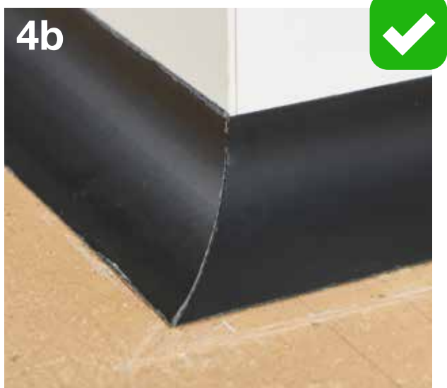
This shows a neat mitre with the cove former cut and fitted at the correct angle.
