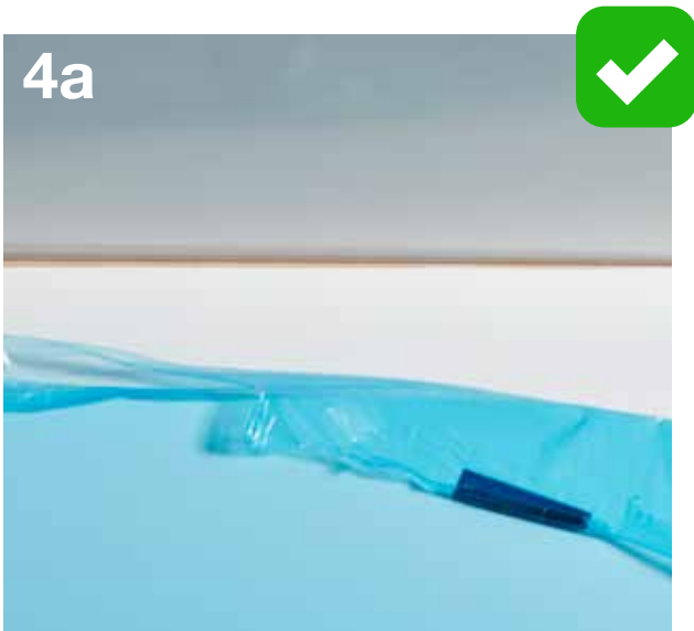
This shows Altro Whiterock joining a ceiling with a 3mm gap.
