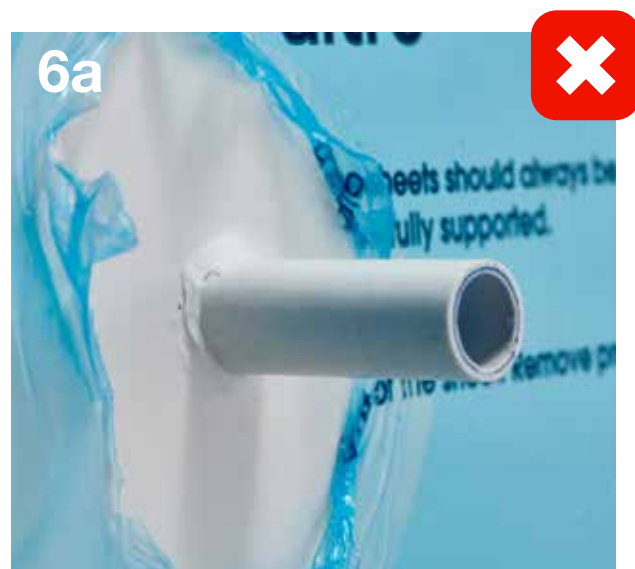
This shows an uneven, thick mastic seal with a gap on one side.
