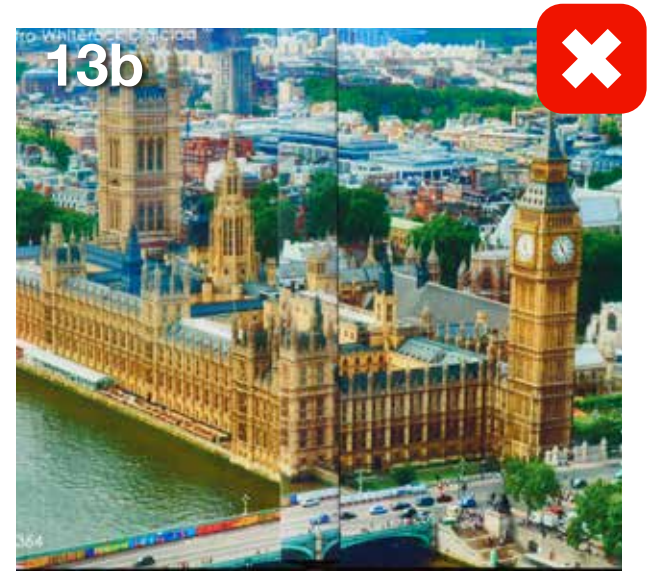
This shows two Altro Whiterock DigiClad sheets installed with a poorly aligned matching trim (take a close look at the bridge!).
